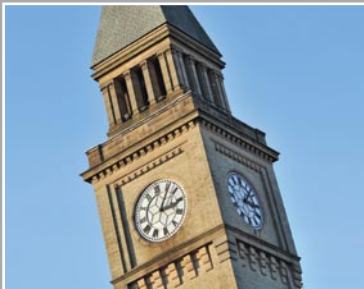
Adjacent Town Hall
